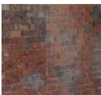
Red and some multi-grain brick with Flemish bond.
