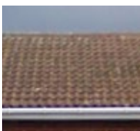
Brown pantiles with white soffits.
