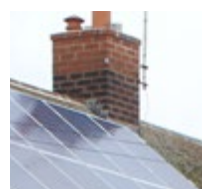
Shared, centrally placed chimney stacks with four pots.
