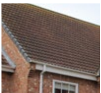
Red and brown pantile roofs, some concrete roof tiles.
