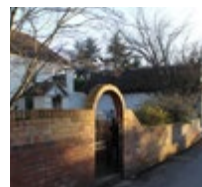
Brick walls with English garden bond, varying in heights but generally 1.2m approx.
