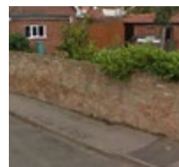
Low walls in red brick with English garden bond.
